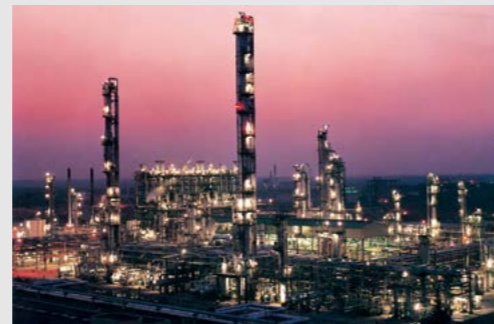
The Zhongyuan Ethylene Project imported by the Company
