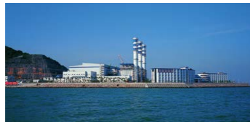
Full view of Qianwan Turbine Power Plant
