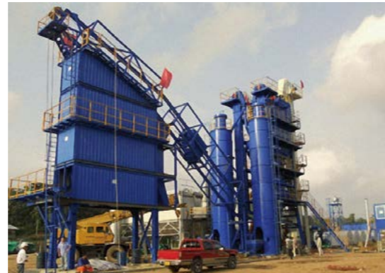
Check on equipment safety performance for Southern Sri Lanka Highway Project
