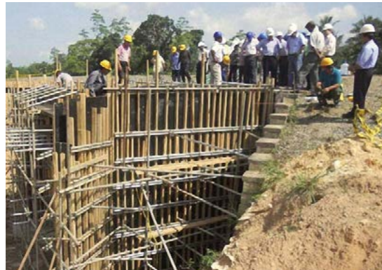
Safety check on the support of construction scaffold at a culvert for Southern Sri Lanka Highway Project
