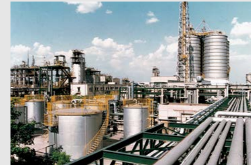
The Polyester Project in Jinan of Shandong Province
